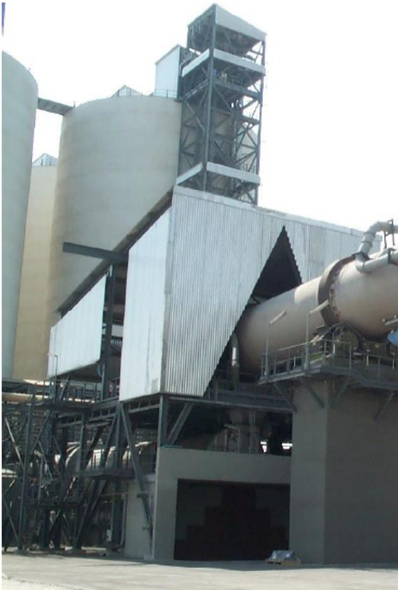
**Picture 2 - Firing Building / Front View with Hot Dump Chamber**
